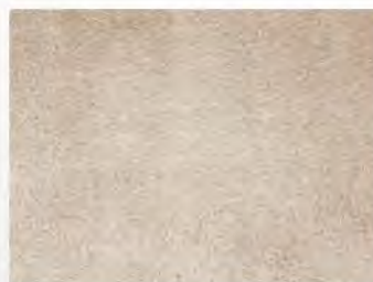
Condition B Blasted to Sa3
