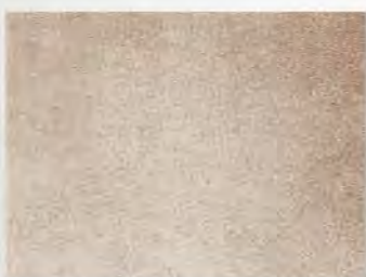
Condition A Blasted to Sa3
