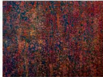
Condition B Blasted to Sa1
