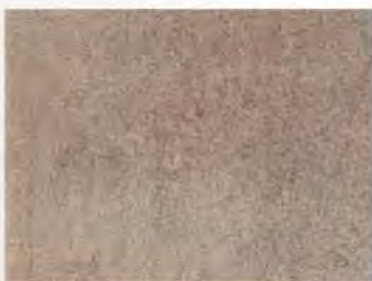
Condition A Blasted to Sa2.5
