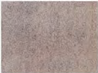
Condition A Blasted to Sa2
