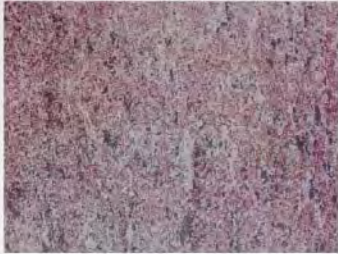
Condition A Blasted to Sa1
